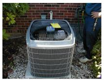
To properly charge a system, add or remove refrigerant until the actual superheat value is within ±5°F of the value obtained from the chart below. If the actual superheat value is higher than what is stated by the chart, add refrigerant to the system. If the actual superheat value is lower than what is stated on the chart, remove refrigerant.
