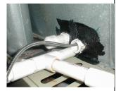
num or its own casing. To leak search this area, a section of the casing surrounding the evaporator must be removed. On some systems this may be a time-consuming task.
